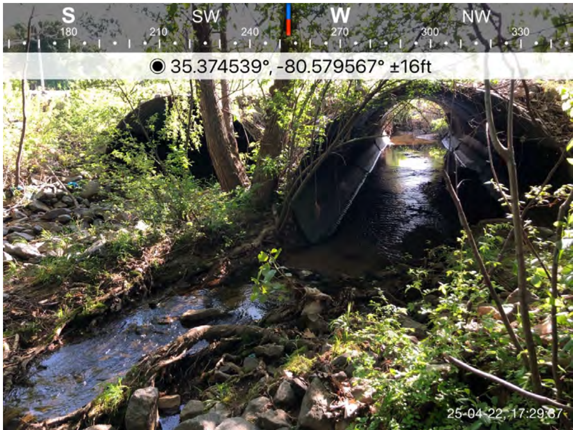
Photograph 3: Existing culvert between borings B-3 and B-4.
